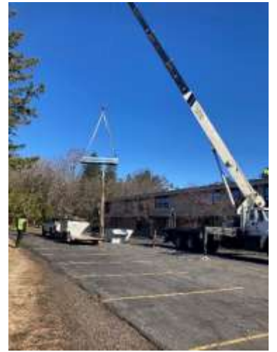
New air source heat pump HVAC system, installed in early May.
