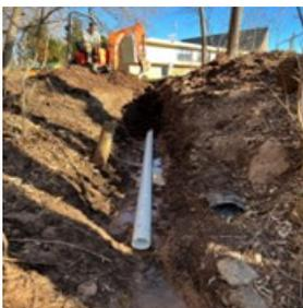
Many thanks to Matt Ryan and Alex Dean who recently dug out the sump pump drain tile and discovered a long length completely clogged with tree roots. The drain now runs freely!
